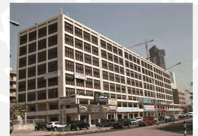
Al Shawafat Complex
