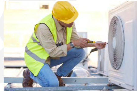
Air conditioning maintenance
